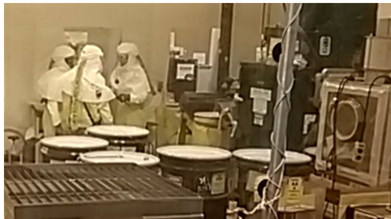
Left: Unloading drums from over-pack drums in WMF-635 tent.
