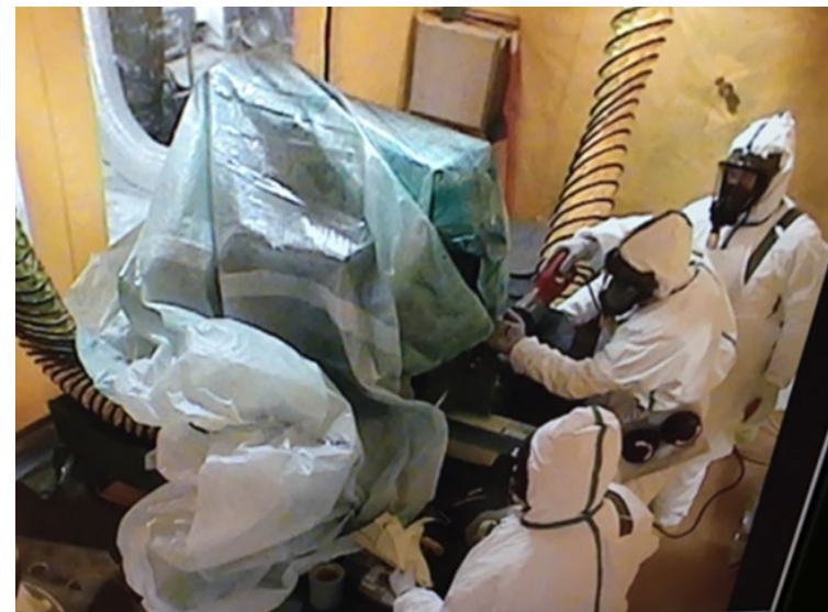
Left: Unloading drums from over-pack drums in WMF-635 tent.
